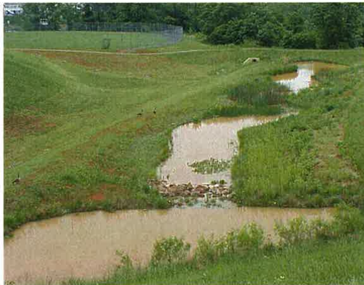
Constructed Stormwater Wetland – becoming stabilized, emergent vegetation barely visible.
