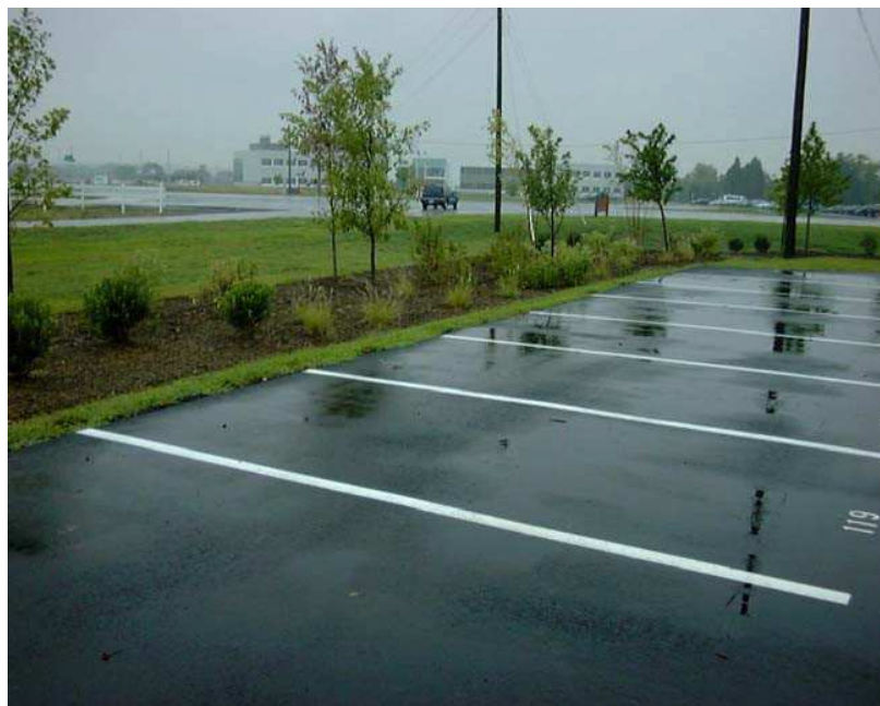
Bioretention Basins in office setting parking lot.
