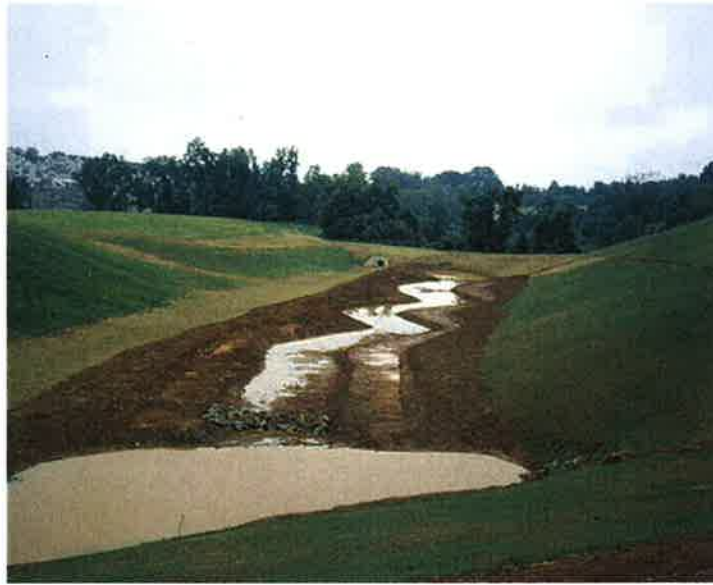
Constructed Stormwater Wetland – recently completed.
