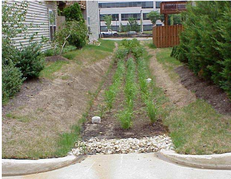
Bioretention Filter in ultra-urban setting. Note curb cut, gravel energy dissipater, and clean out/observation wells.
