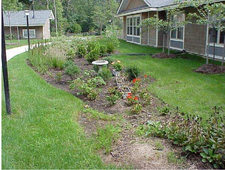
Bioretention Filter in multi-family residential setting.
