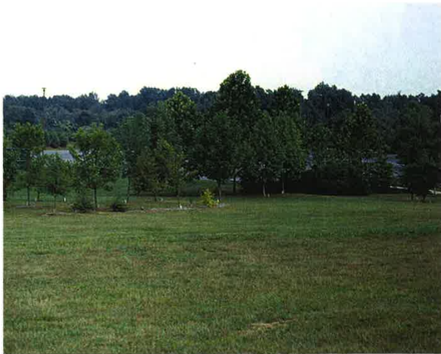
Vegetated Filter Strip. Note landscaped areas parallel to contours to force runoff to spread out. No evidence of channel flow short circuiting filter strip.
