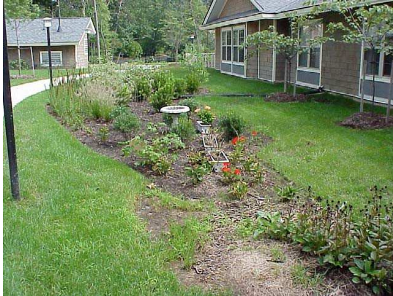
Bioretention Filter in multi-family residential setting.
